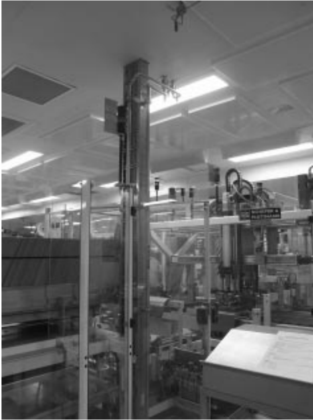
Fig. 15.5 Walkable ceiling with integrated luminaires above the conditioned production zone H and a vertical cable trunk to the machine.
